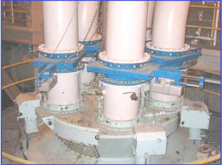
Actuated Coal Flow Balancing Damper
